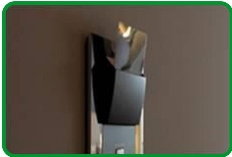
In order to avoid this problem, smarter key card holders can be installed that both identify the key card and also manage a set-back position for the temperature
